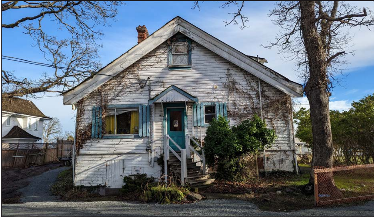
Fig. 25: Annandale from the west, 2023. This is technically the “back” of the property. (Source: Cummer)
