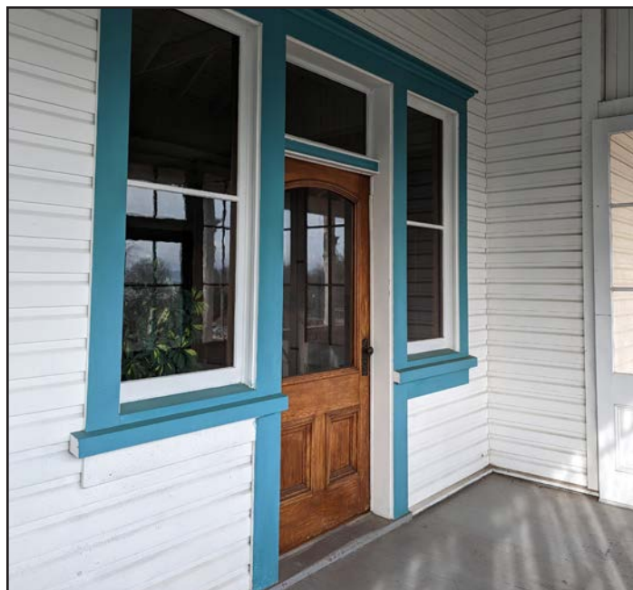
Figs. 41 to 42: (Top) Example of the numerous surviving original double-hung horned wood windows, 2023, in largely good condition. (Bottom) Original front door of Annandale, 2023, also in good condition. (Sources: Cummer)
