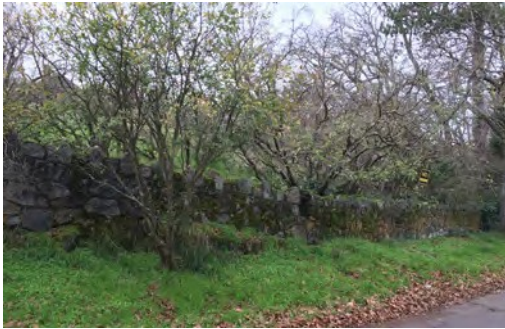
Prospect Place stone wall with natural vegetation.
