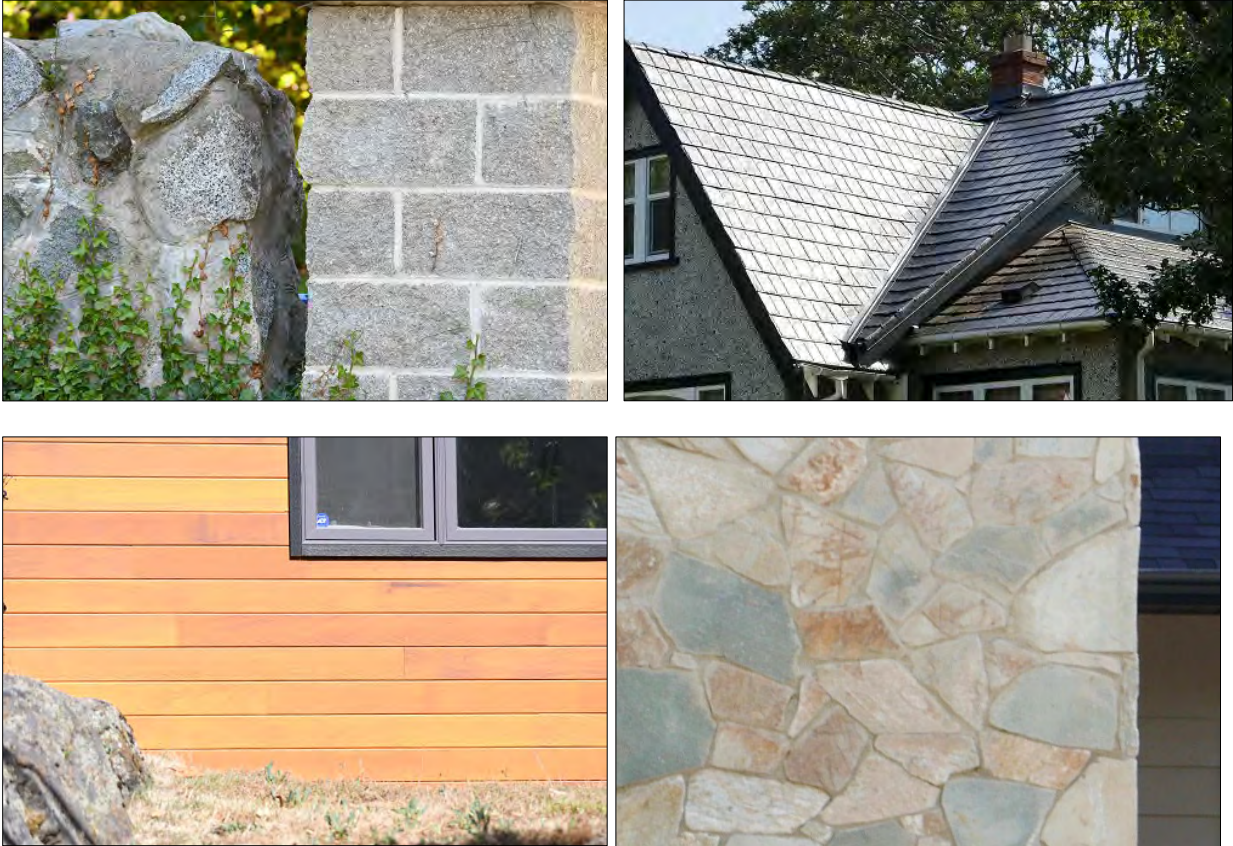
Examples of imitative modern materials and finishes that are not recommended for new construction in The Prospect.
