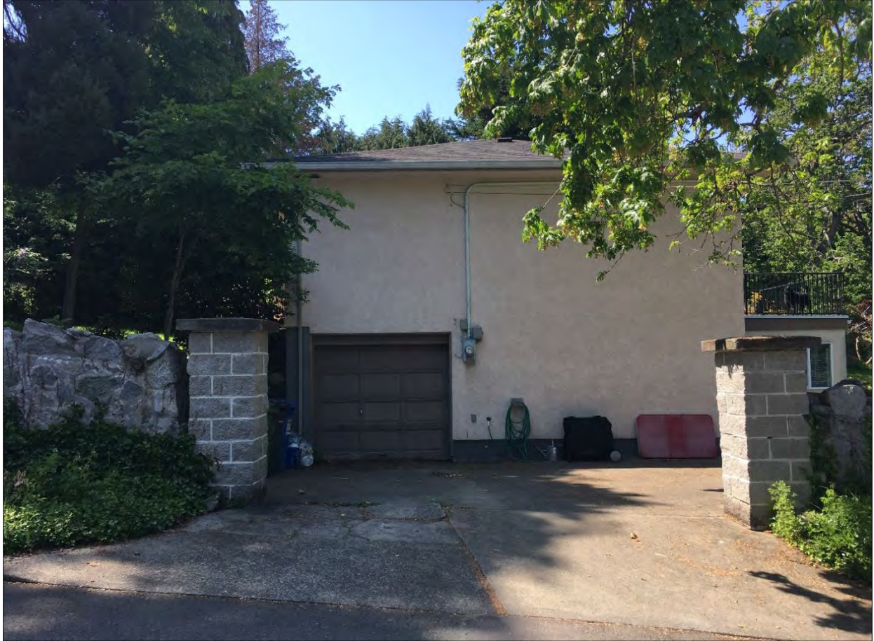
Example of inappropriate form, scale and massing (also demonstrating incompatible building materials, incompatible landscaping materials, an expansive and impermeable driveway and inappropriate door and window design).
