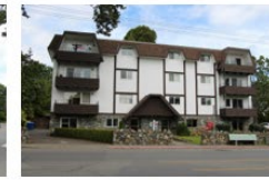
ADJACENT EAST PROPERTY FROM OAK BAY AVENUE
