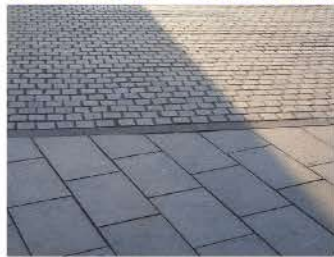
Ensure pathways + surfaces are accessible for all; use asphalt, poured concrete, compacted crushed gravel, or unit pavers to define spaces
