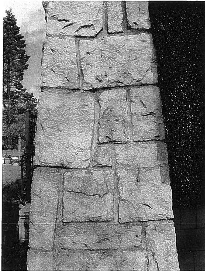
Detail of granite pier with grey mortar
