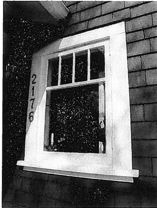
Original wood frame casement window on front elevation
