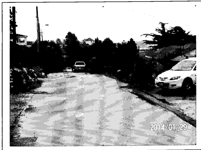
2). Existing road surface at #157 - #175, #158 - #176 Barkley Terrace
