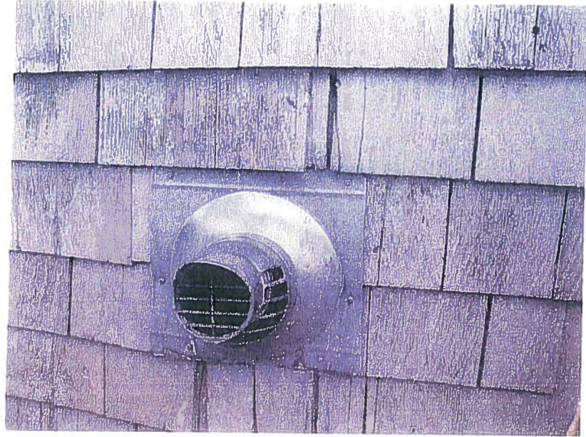
Detail of shingle siding. Note shingles that are cracked and weathered. These should be replaced in kind.
