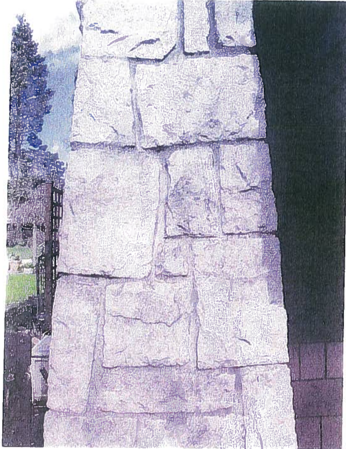
Detail of granite pier with grey mortar
