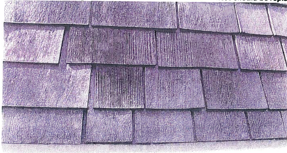
Detail of shingle siding. Note shingles that are cracked and weathered. These should be replaced in kind.
