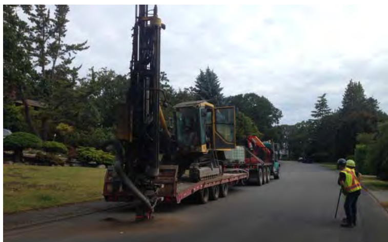
Western Grater rock probing along Norfolk Road.
