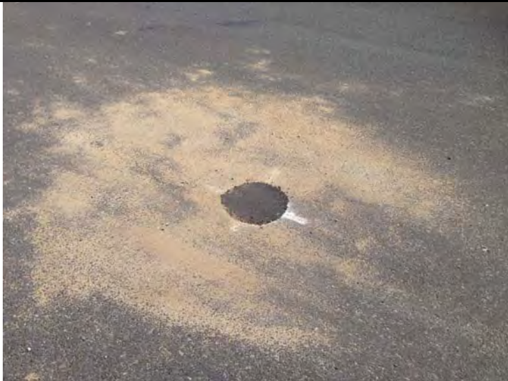
Completed asphalt borehole patch at BH16-07.
