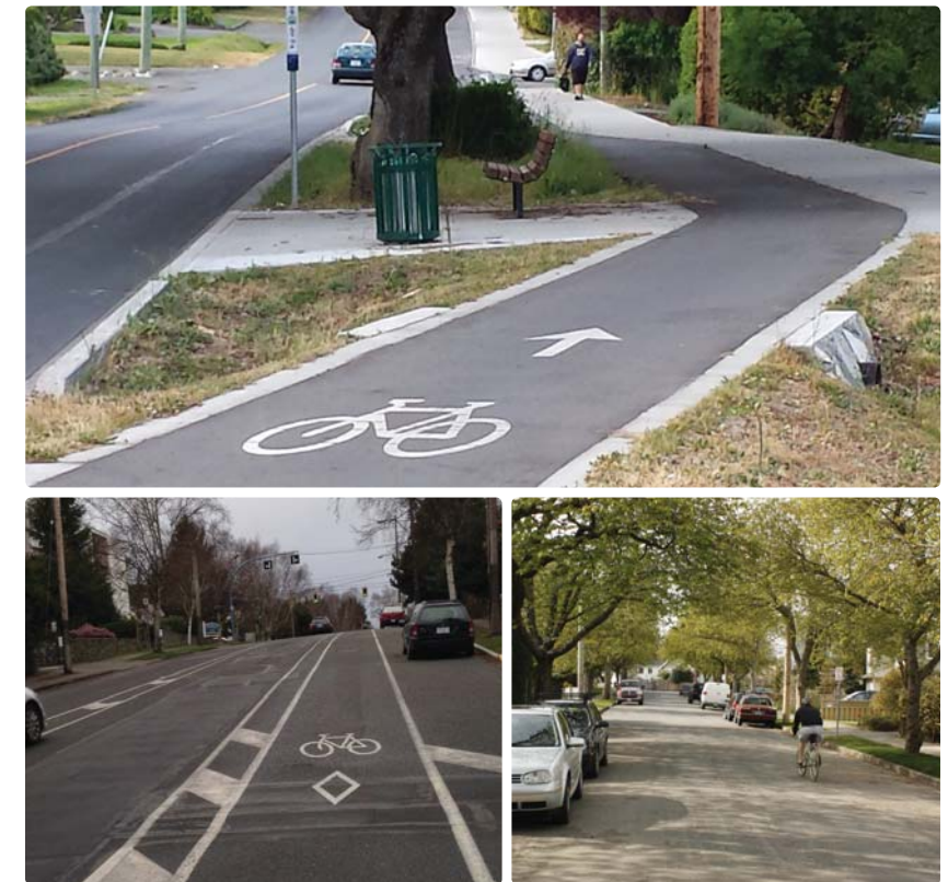
Examples of bicycle facility types include a fully separated lane (i.e. "cycletrack") at top, a bike lane separated from vehicles by a "buffer" area at bottom-left, and a neighbourhood bikeway where cyclists share the street with vehicles on identified low volume routes.
