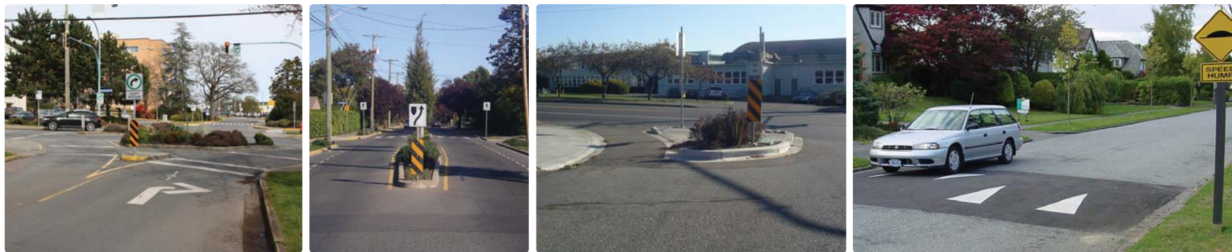
Examples of various traffic calming features (from left to right) - A Right-in, Right-out Island on Richmond Road at Royal Jubilee Hospital, a Centre Median on Finlayson Road, a Directional Closure on Hillside Avenue, and a Speed Hump.
