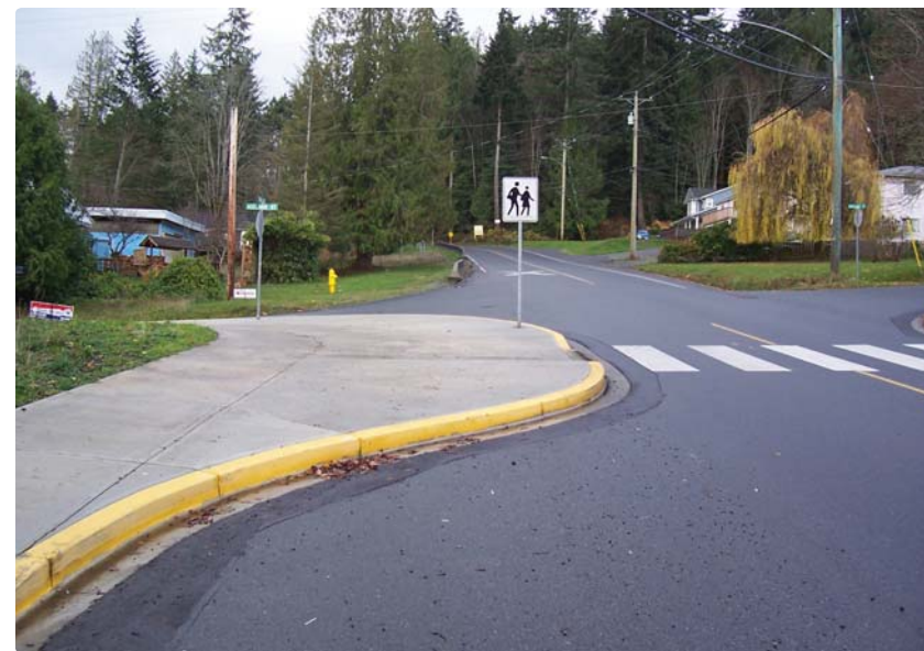
Sample image of a curb extension that reduces the pedestrian crossing distance and manages vehicle turn speeds
