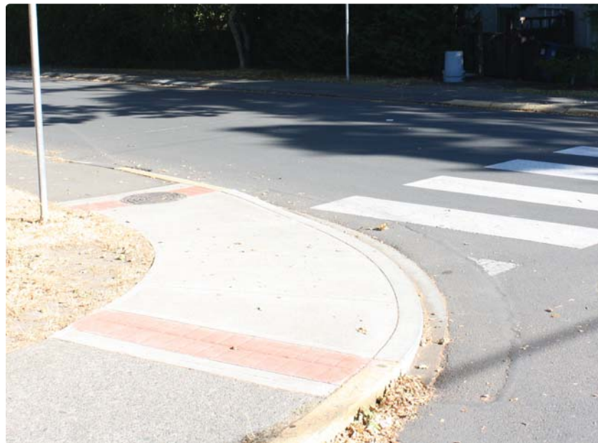
Sample image of the District's standard curb ramp and tactile strip placed at pedestrian crossing locations
