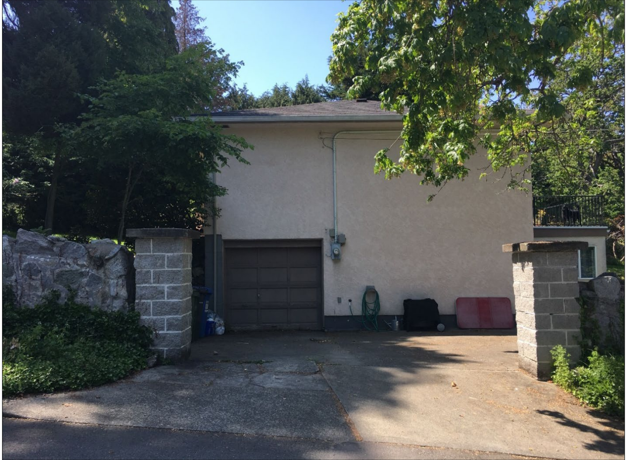
Example of inappropriate form, scale and massing (also demonstrating incompatible building materials, incompatible landscaping materials, an expansive and impermeable driveway and inappropriate door and window design).
