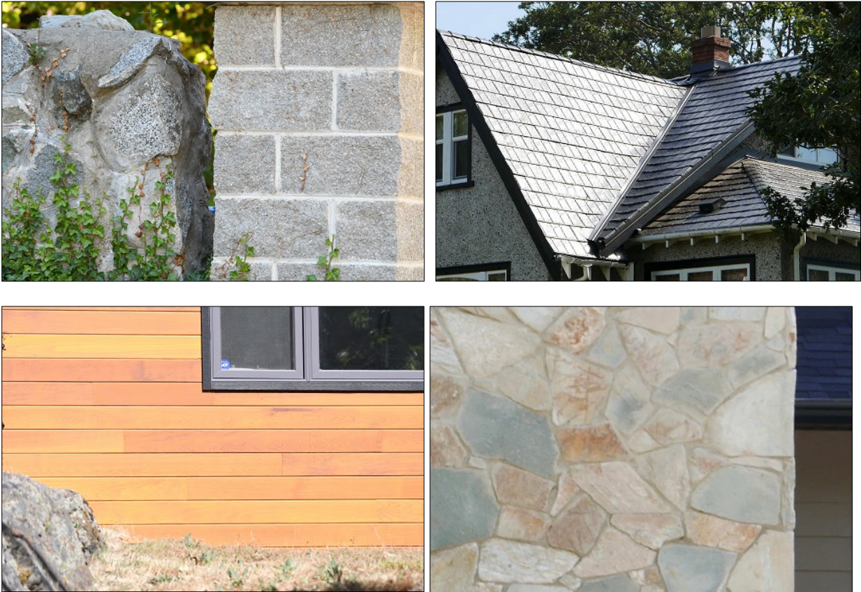
Examples of imitative modern materials and finishes that are not recommended for new construction in The Prospect.
