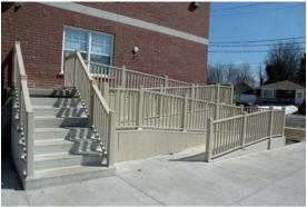
A bicycle stairway channel (left) and wheelchair accessible ramps (right) are examples of features that can be built into staircases to better accommodate bicycle and wheelchairs.
