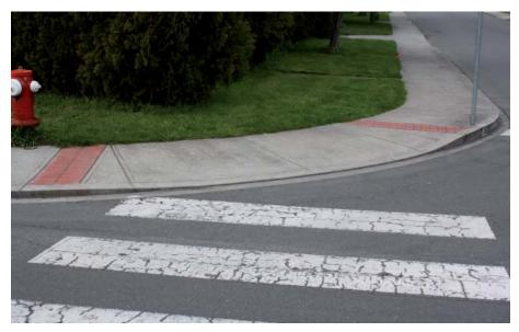
Example of recent curb ramp improvements in Oak Bay aimed at ensuring an appropriate slope and tactile warning strips that identify the crossing point.
